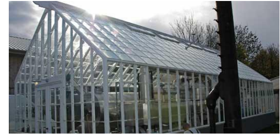
Greenhouse, boiler, biochar Stirling Engine (DK)
