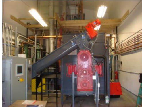
3 MMBtuh Hot Water 25% Char+Ash
