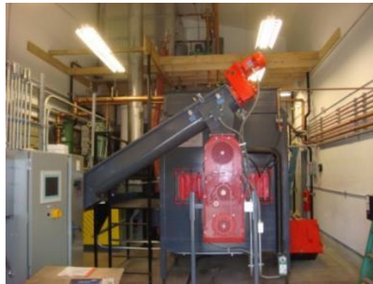
Boiler 3 MMBtuh Hot Water 500 lb/h 25% Char
