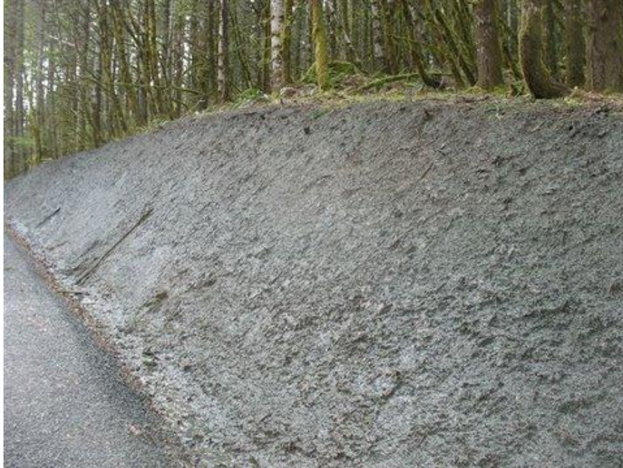
Jory clay cut slope where nothing had grown for 10 years.
