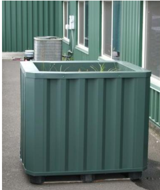
A roof drain tote built for zinc removal
