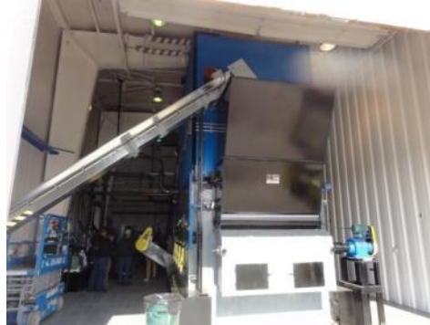
THERMAL OIL HEATER 10 MMBtu
