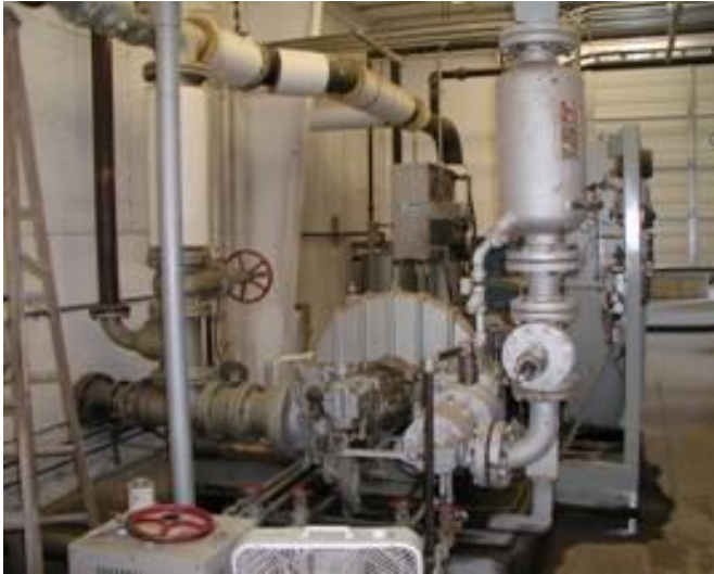
500 kWe Back Pressure Turbine NH
