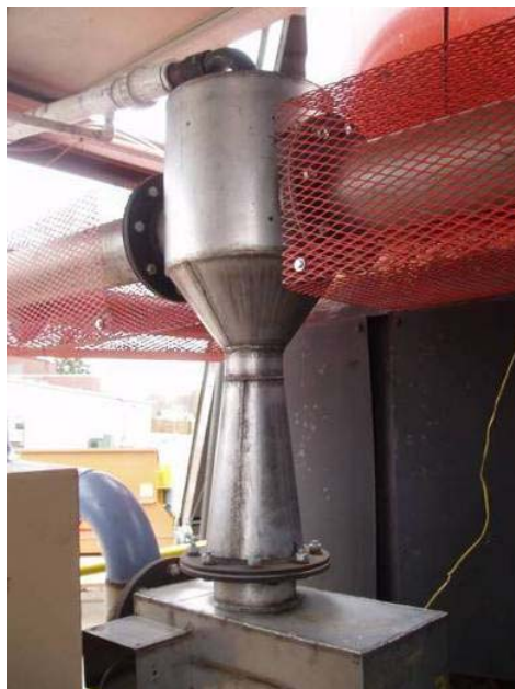
GAS IS COOLED AND CLEANED WITH A WET VENTURI SCRUBBER AND DRY FILTERS
