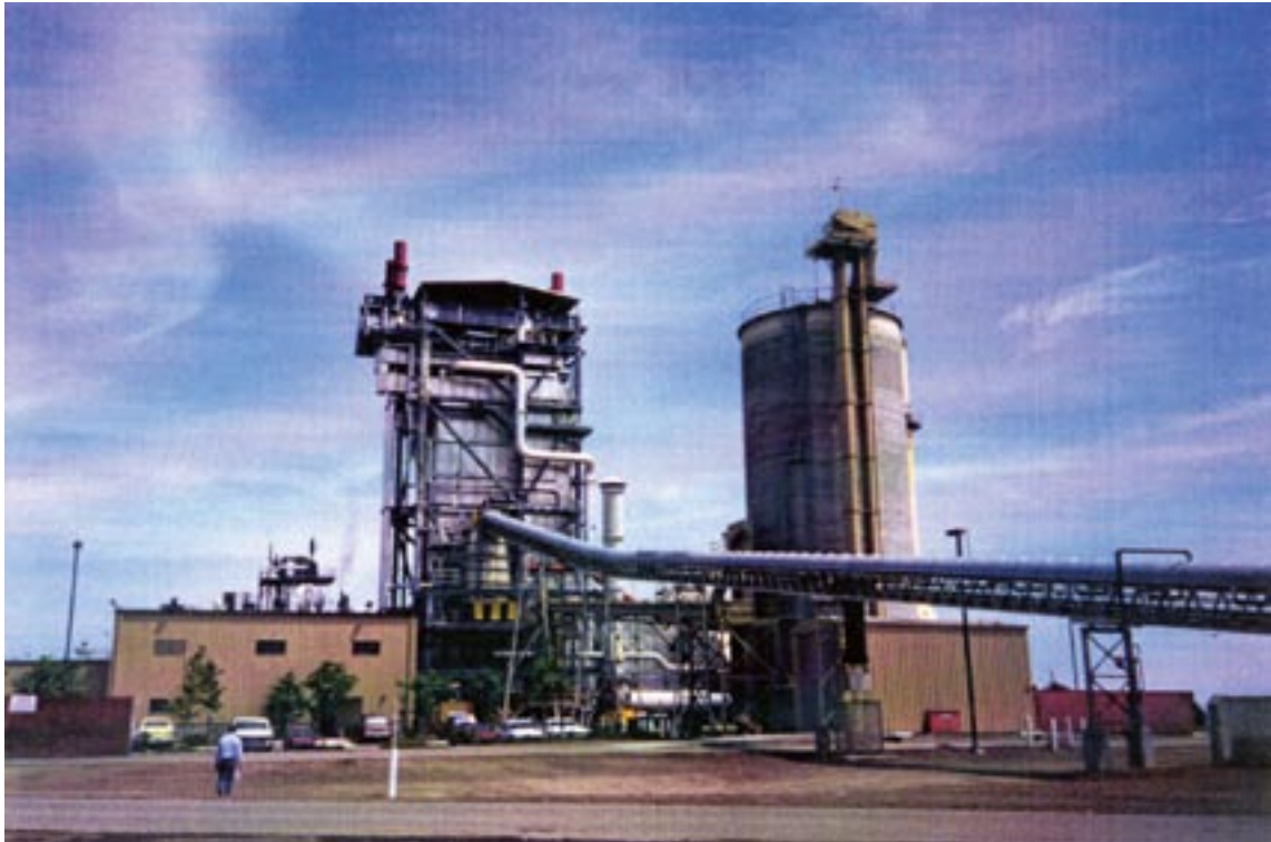
Figure 5 CFB-1 Circulating Fluidized Bed, 25 MWe, Woodland, CA
