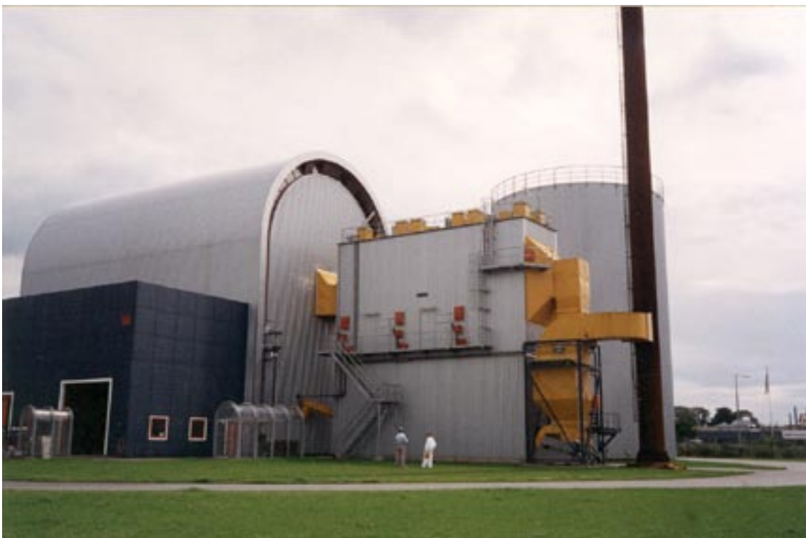
Figure 3 Grate-3 Straw fired moving grate CHP 5 MWe, Slagelse, Denmark
