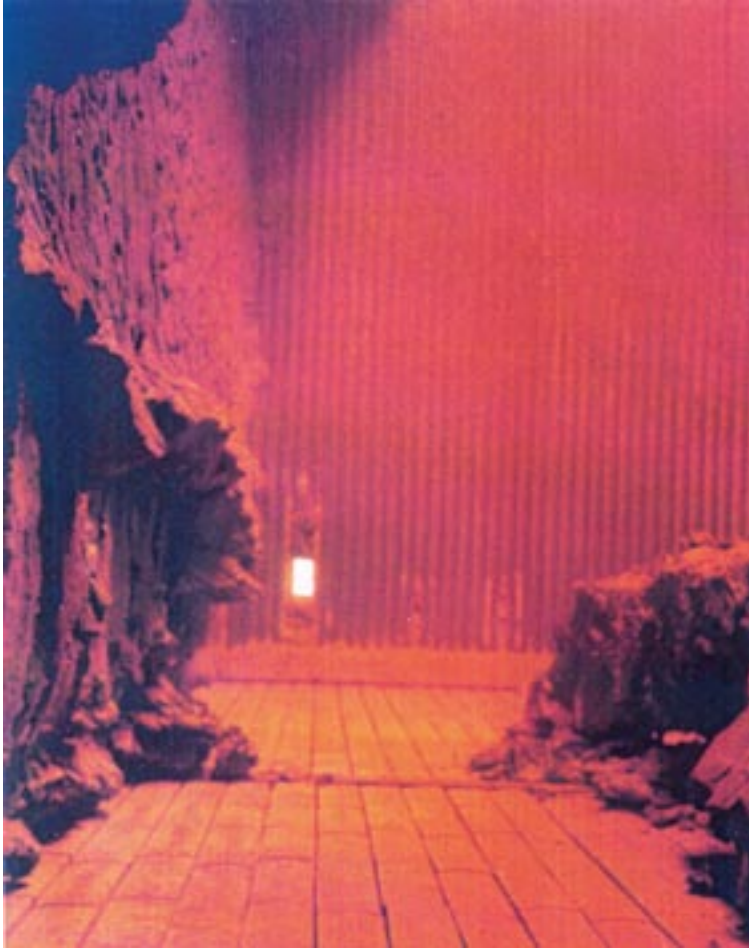
Figure 7 Slagging on wall after four days of burning a high percentage of Urban Tree Trim-mings in Grate- 1. Deposit that fell from the wall is 3' high and 14' long. 4 days operation. (Hydra Co. 1992)
