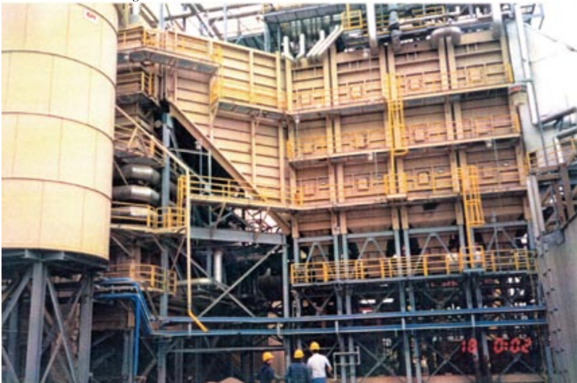
Figure 6 FBC-1 Bubbling Fluidized Bed, 25 MWe, Delano, CA
