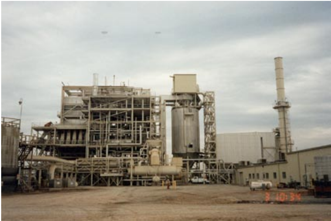
Figure 2 Grate-1. Spreader stoker with traveling grate, 20 MWe, Imperial, CA
